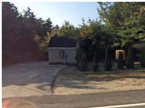
Figure 7 – FairPoint Communications remote terminal on Main St. in Jaffrey. Note the yellow generator to the right. Photo credit: Google Street View. A town may be provided service from a central office in a neighboring town.
